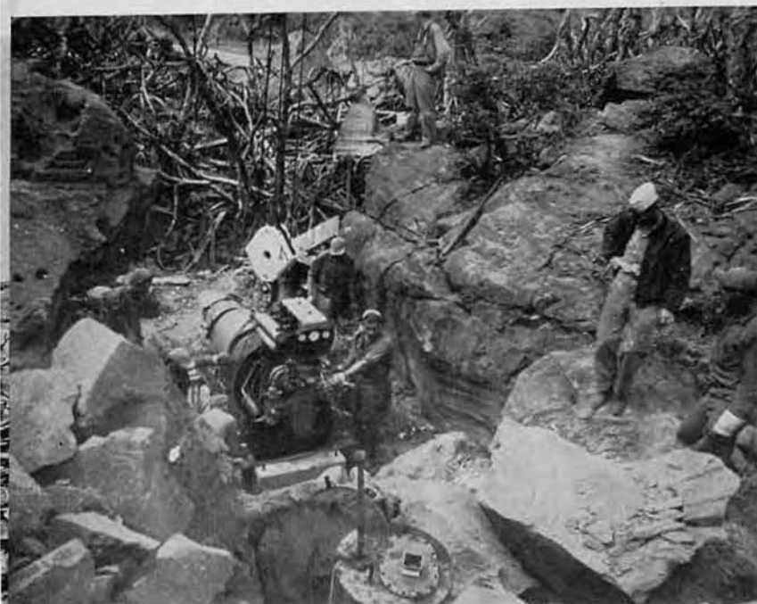
Installing a Jap Generator.
