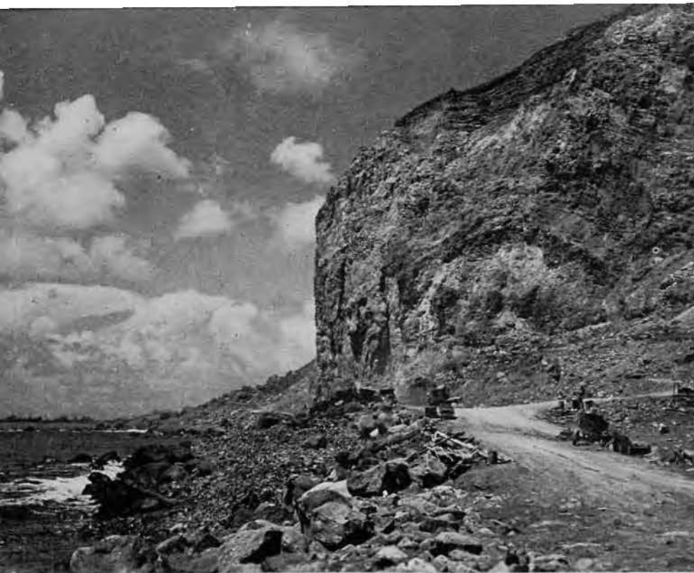
Blasted From Here.
