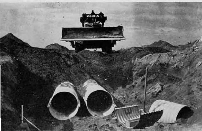
Completion of Drainage Project.
