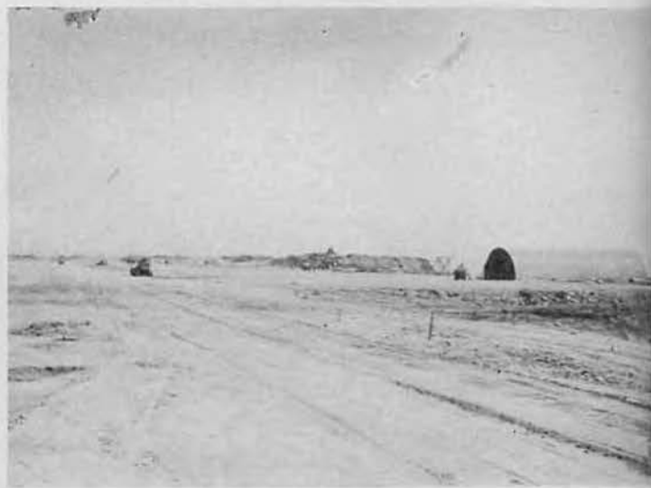
Progress on Our Parkway.
