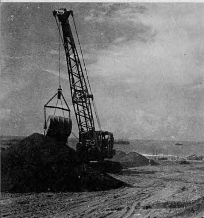
Dragline Digging Drainage Ditch.
