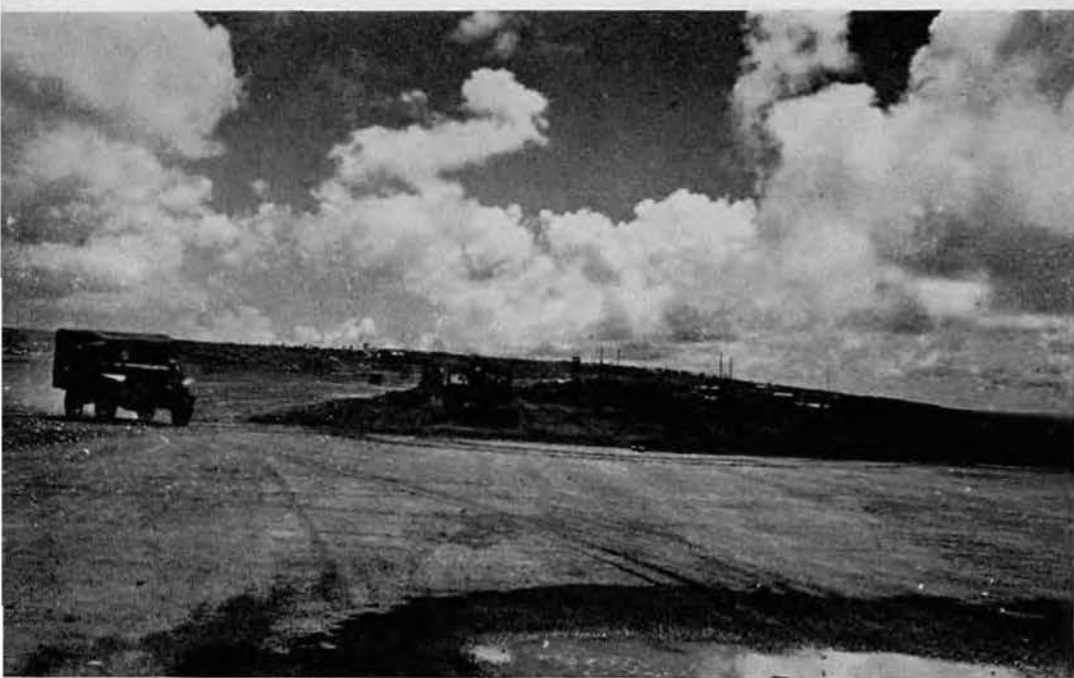
Parking Area Under Construction
