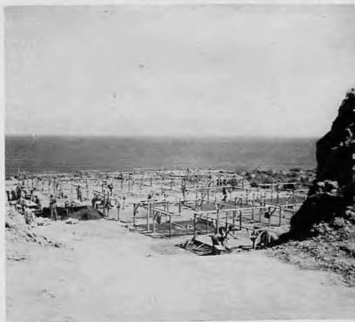
Tent Frames and Concrete Decks for Co. B.
