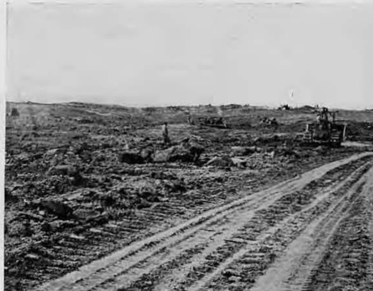
A Dent is Made in the Airstrip Site by Dozers, Tournapulls, Carryalls, Trucks, Men.
