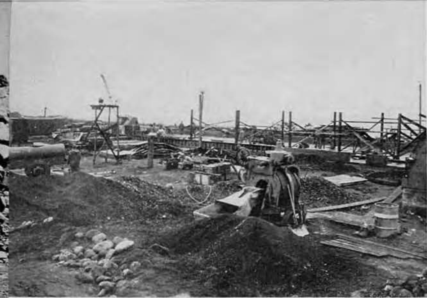
New Galley Under Construction.
