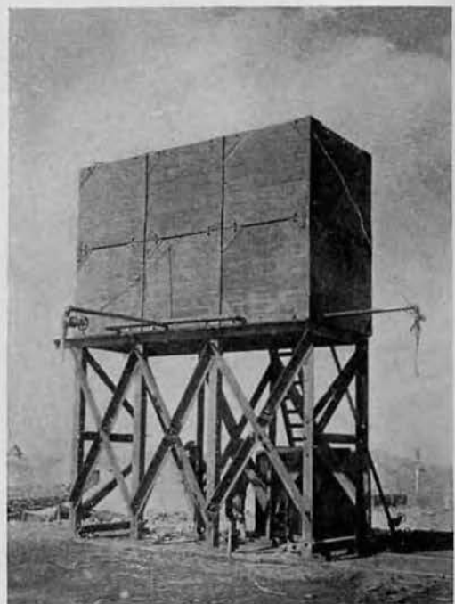
Pontoon Water Tanks.
